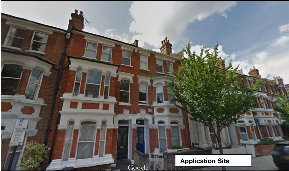
Photo 3: Existing front elevations along Calabria Road
