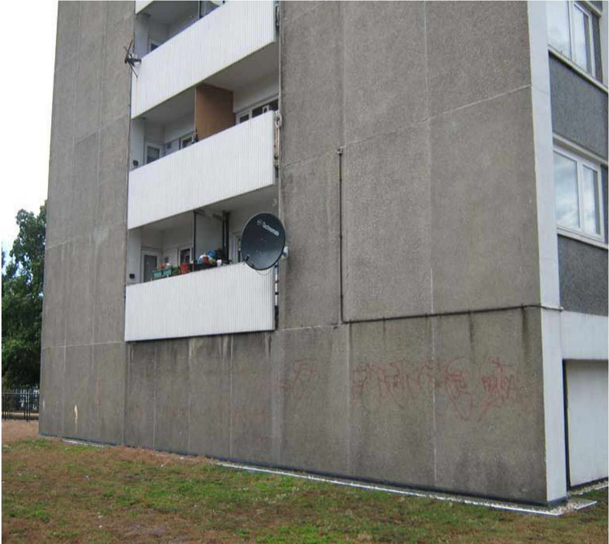
Image 1: Ground floor side elevation of Michael Cliffe House facing south
