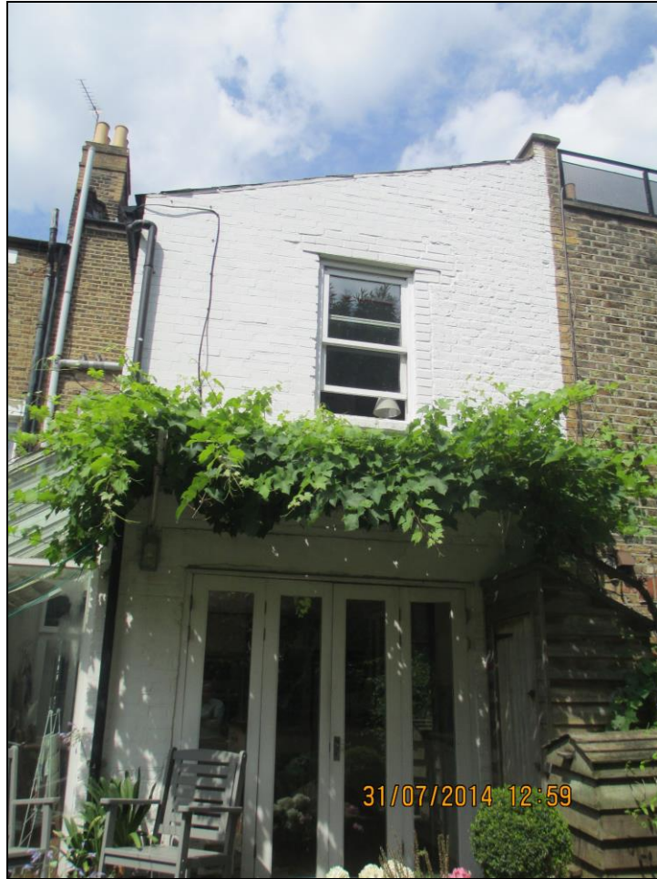
Image 3: View of existing rear elevation of 48 Melgund Road
